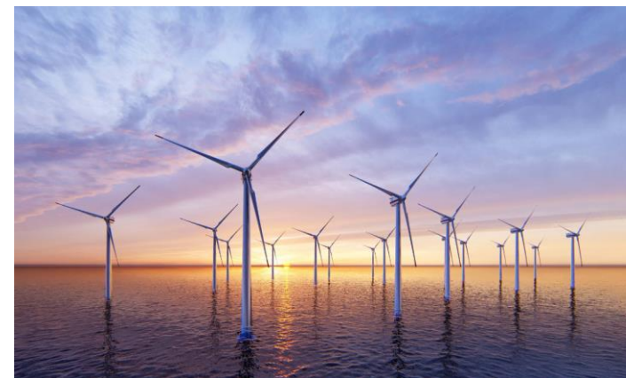
Offshore Wind Farm
